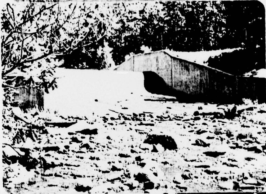
Spillway Looking Upstream
