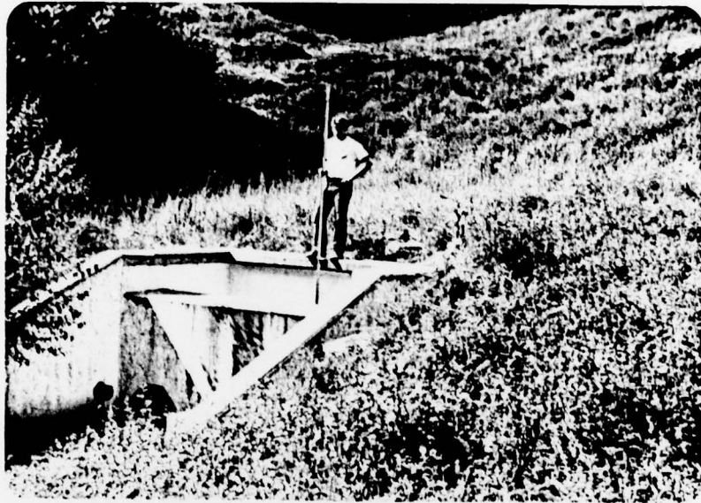
C. Main Spillway Impact Basin
