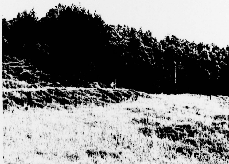
F. Embankment Extension Along Right Side of Auxiliary Spillway Exit Channel
