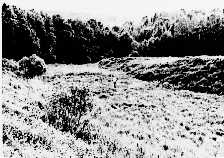
E. Auxiliary Spillway Exit Channel
