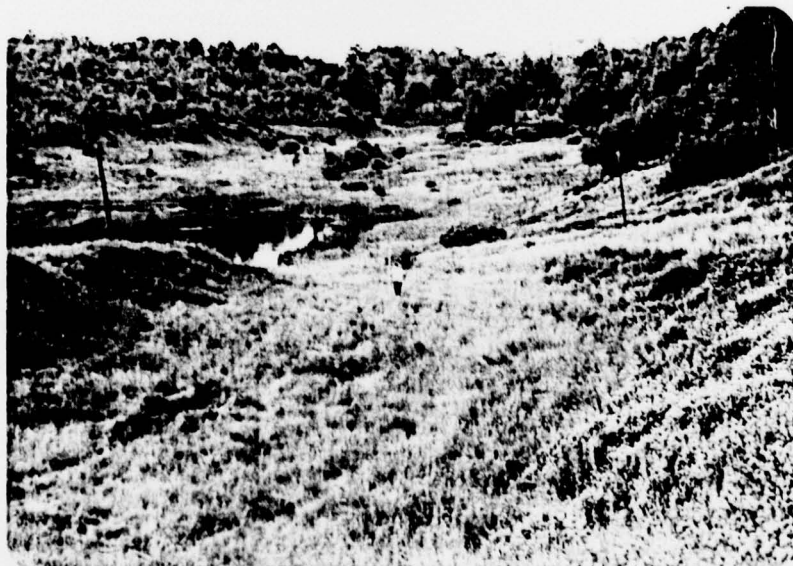
D. Auxiliary Spillway Approach Channel
