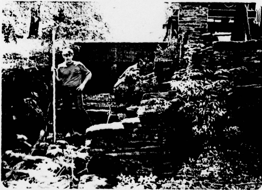
D. Dry Masonry Structure at Spillway.
