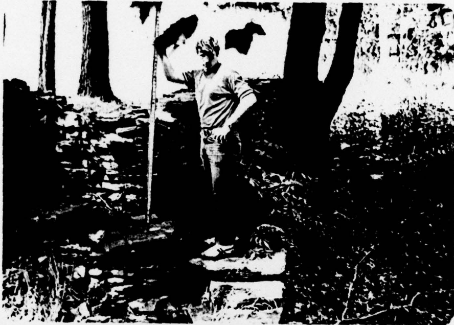
C. Dry Masonry Structure at Left Abutment.
