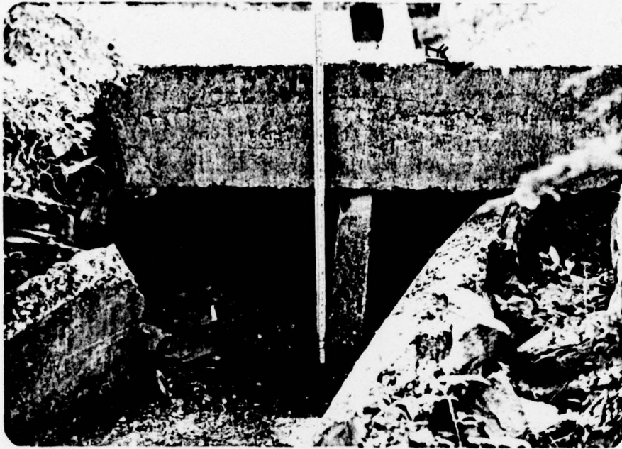
J. Spillway Box Culverts at Downstream End.
