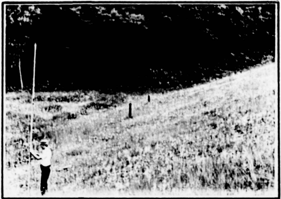
Monitors on downstream slope near right abutment.
