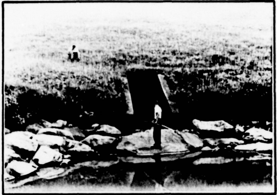
Discharge end of outlet works.
