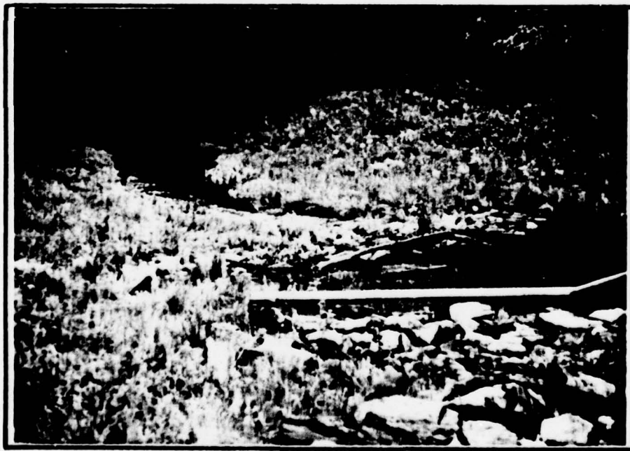
Immediate downstream exposure. Note perforated metal underdrain pipe.
