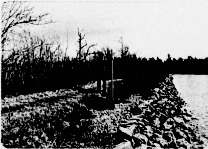
B. Upstream Slope
