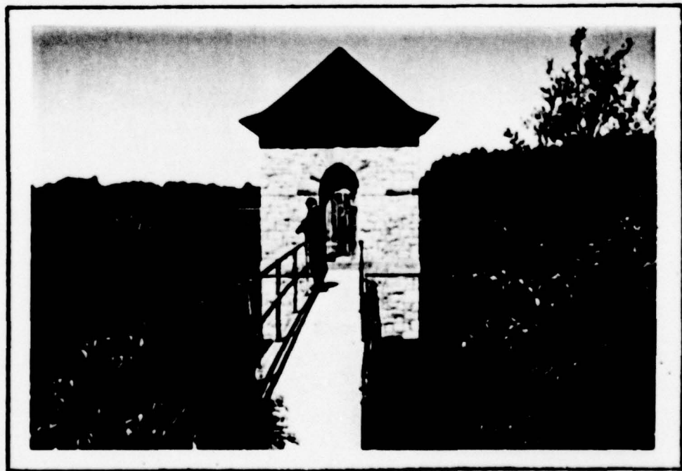
CATWALK AND GATEHOUSE WITH BROKEN RAILING ON THE RIGHT SIDE OF THE CATWALK
