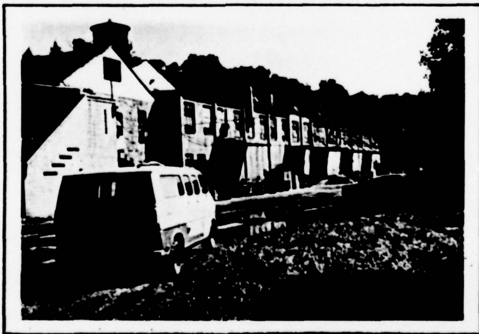
POTENTIAL DAMAGE AREA APPROXIMATELY 2,000 YARDS DOWNSTREAM OF THE DAM
