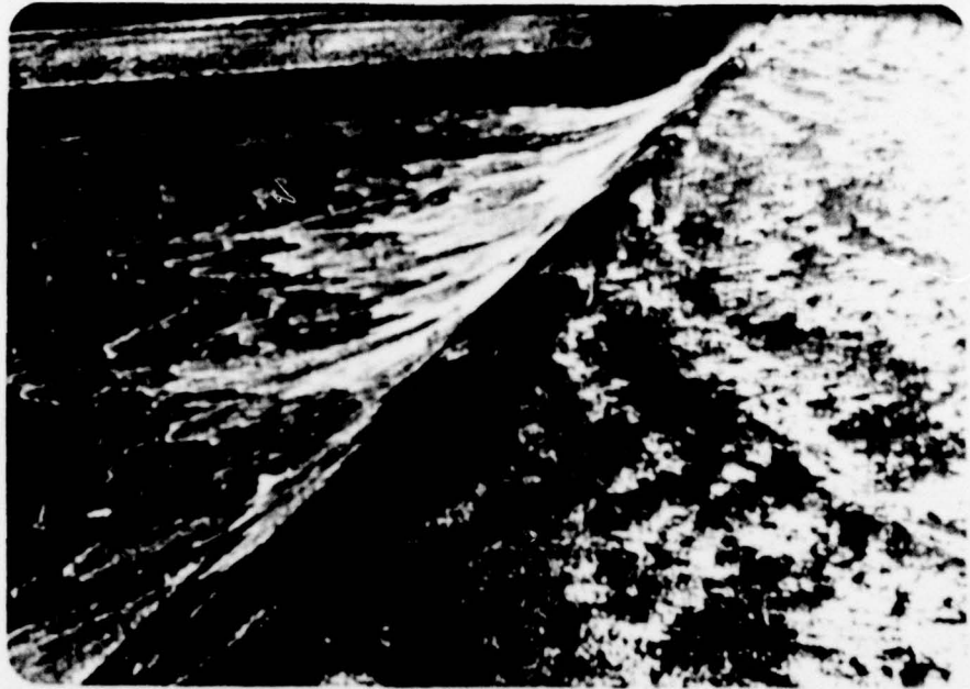
Photograph No. 3 Spillway crest.
