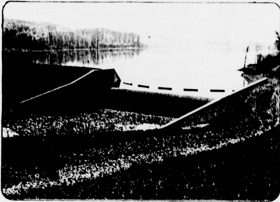
PHOTO 1. View of Spillway and Reservoir from Left Abutment Hillside
