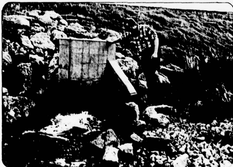
PHOTO 6. Head Wall for 12 inch A.C.C.M.P. from Stilling Basin
