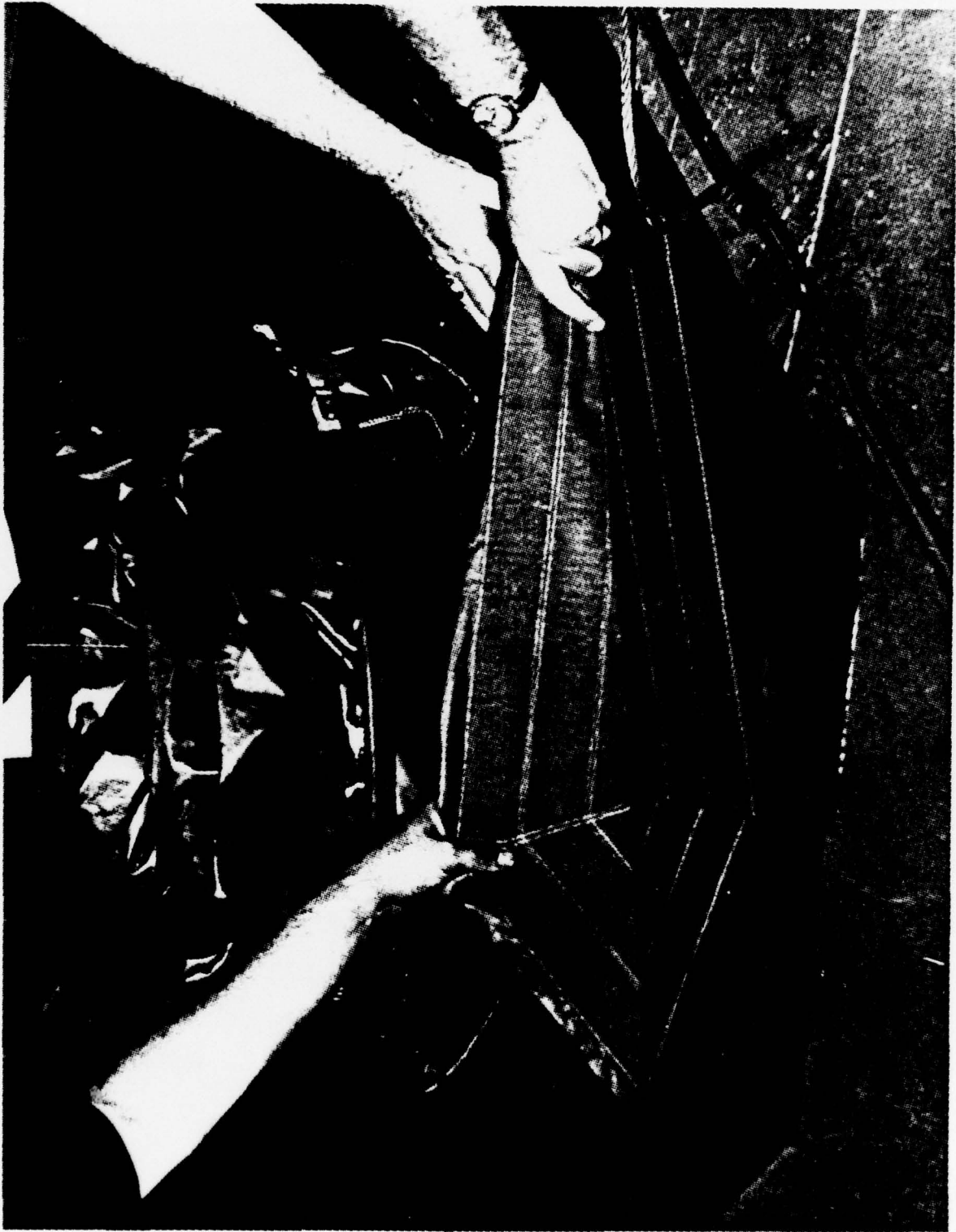
FIGURE 16. VRD SKIRT AND HOOP OVER TANK OPENING 35
