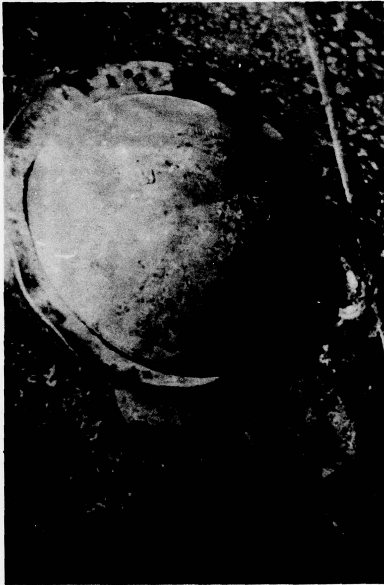
Figure 23. Closeup of button anode at Cordell Hull showing blistering of vinyl paint (Nashville District).
