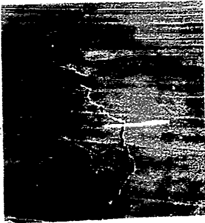
Photograph 11. Crack No. 2 on runway location after routing with 1/2-in.-diameter bit.
