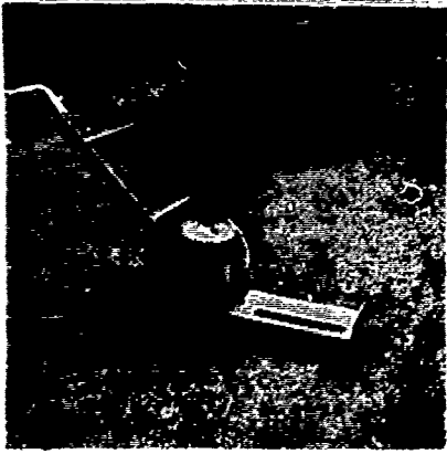
Photograph 9. Infrared heater used for heating interior of prepared groove and surrounding pavement prior to pouring of the sealing materials.
