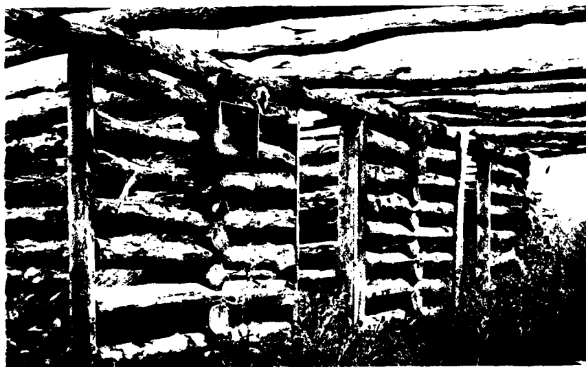
Fig. 17: Interior view of northwest pens through the runway of Building 2, Tract 237. Note saddle notching and door framing of the pens.
