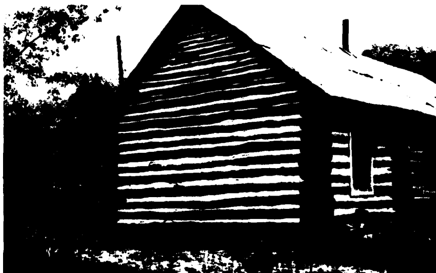
Fig. 66: Back (northwest) wall of Carter Chapel.
