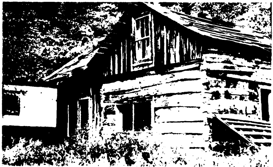
Fig. 93: Southeast wall of log portion of dwelling on Tract 1014. Contrast gable construction with that on opposing wall.
