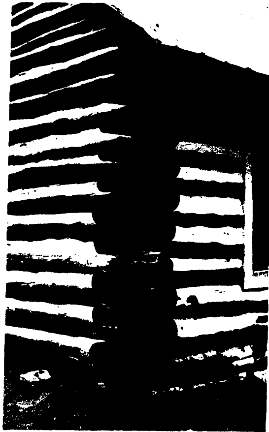
Fig.-67: Detail of saddle notching on logs of Carter Chapel.
