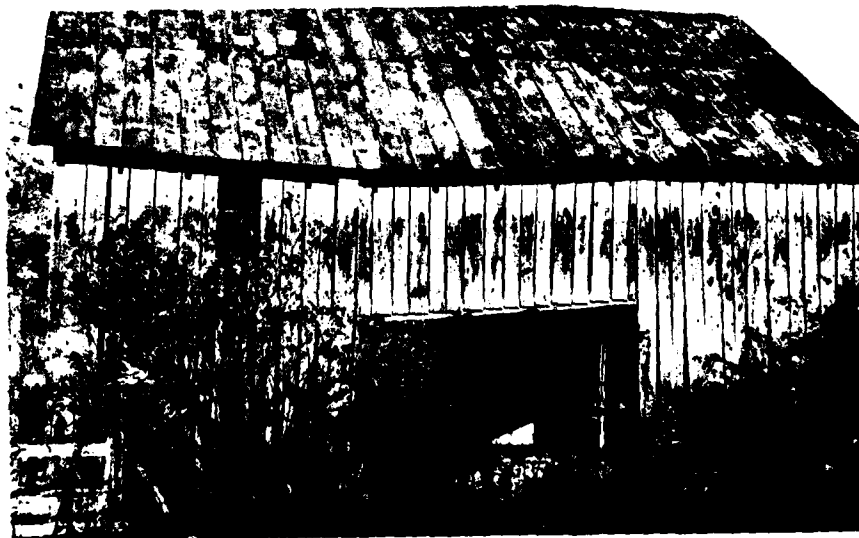
Fig. 83: General view of southwest wall of Building 2, Tract 921. Note runway and use of board rafters.
