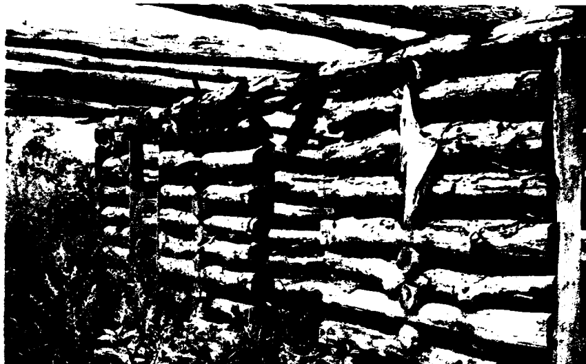
Fig. 16: Interior view of southeast pens through the runway of Building 2, Tract 237. Note saddle notching.
