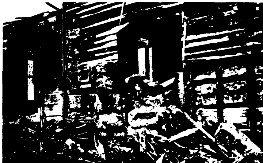
Fig. 40: Collapsed sandstone chimney on western side of dwelling on Tract 404. Note addition at left and use of wood siding over logs.
