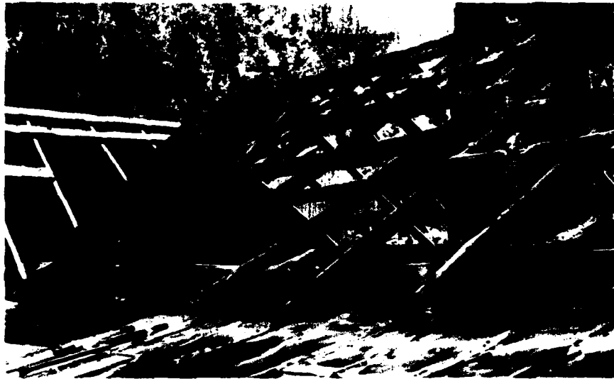
Fig. 76: Detail of roof construction Building 1, Tract 921, looking south. Note the use of decorticated pole rafters over the log portion of the dwelling in distinction to the board rafters over the frame addition (Room 3) at left.
