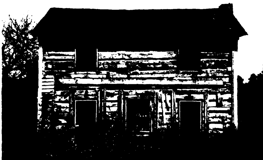
Fig. 21: Main entrance to log home on Tract 239 in southwest wall. Note original door width and remnants of frame siding.
