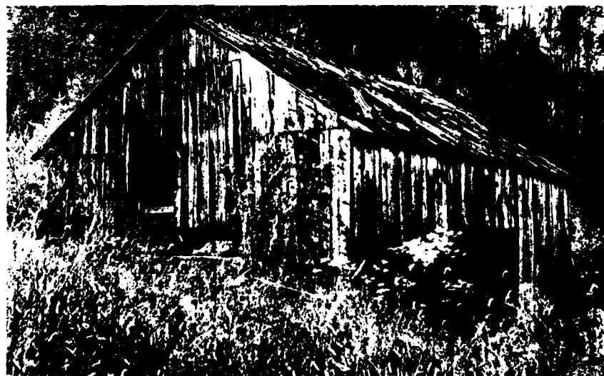
Fig. 81: General view of combination frame and log barn, Building 2, Tract 921 northeast and southeast walls. Note logs in southeast wall.
