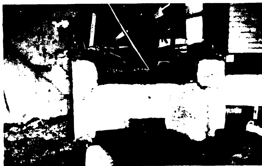
Fig. 55: Building 1, Tract 411. Collapsed cinder block closed sandstone fireplace in northeast wall of Room 1. Note use of frame construction in this wall of the house after removal of the original logs.
