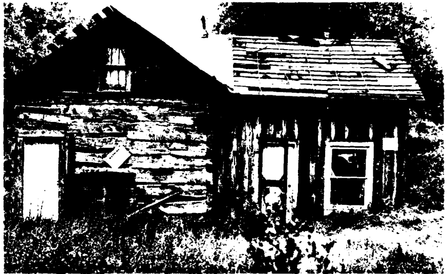
Fig. 92: Northwest wall of log portion of dwelling on Tract 1014. Note former chimney opening and use of riven weatherboards over interstices of some of the logs. Gable is assembled with cut nails.
