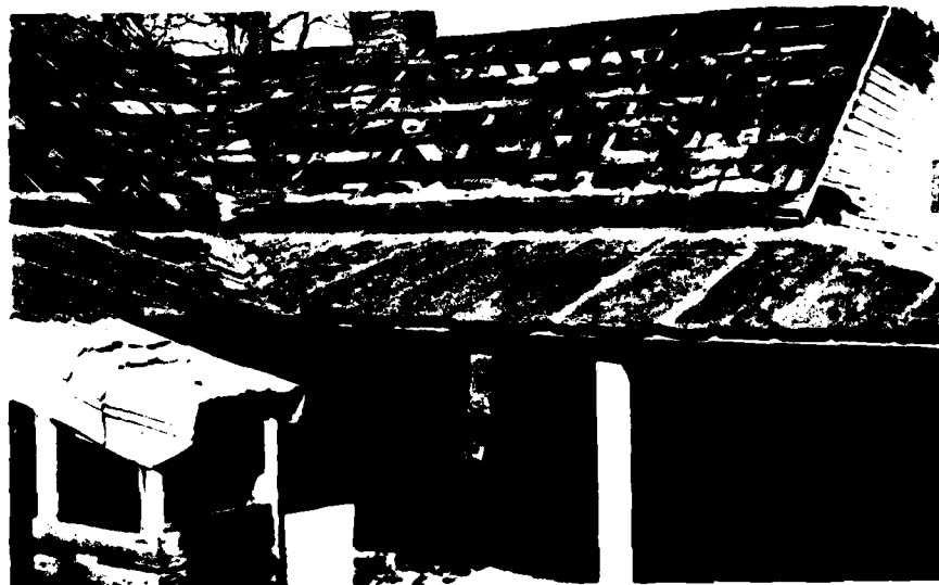
Fig. 77: Detail of porch additions to southwest and southeast walls Building 1, Tract 921. Note frame well head at left.
