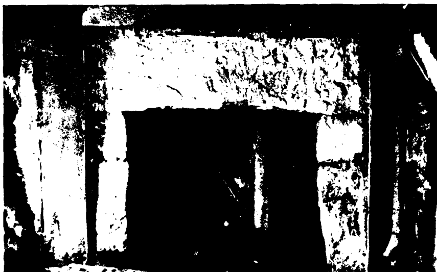
Fig.32 : Detail of dressed sandstone fireplace northwest wall of Building 1, Tract 301. Note whitewash and brick and stone backing.
