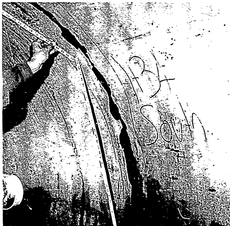
Photo No. A-11 Minor joint spall at Sta. 1+34.
