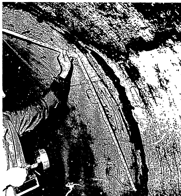
Photo No. A-12 Minor joint spall at Sta. 0+94.
