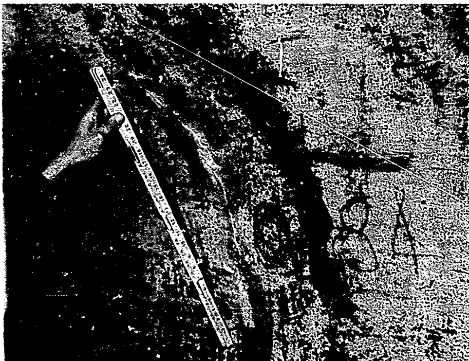
Photo No. A-13 Minor crack sealed by calcium deposits at Sta. 0+84.
