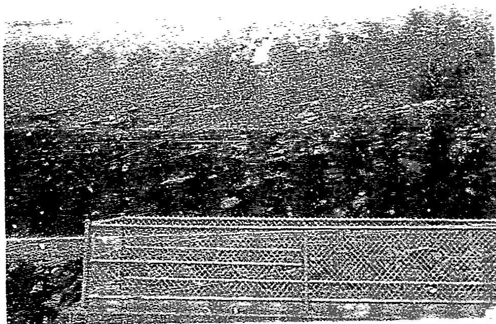
Photo No. 8 Eroding of overburden down to bedrock - right bank above outlet works.
