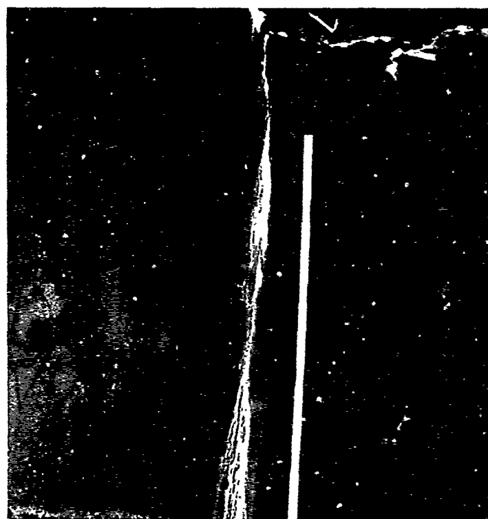
Photo No. B-8 Vertical cracks in North Chamber at Sta. 0+27 sealed by calcium deposits.
