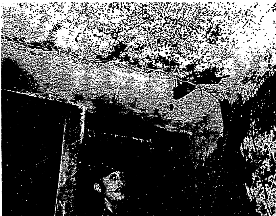
Photo No. A-14 Ceiling cracks in South Chamber sealed by calcium deposits at Sta. 0+67 to 0+69.
