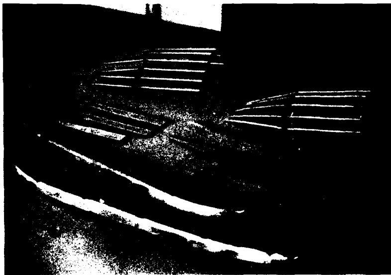
Figure 1. Ice deflectors before installation.
