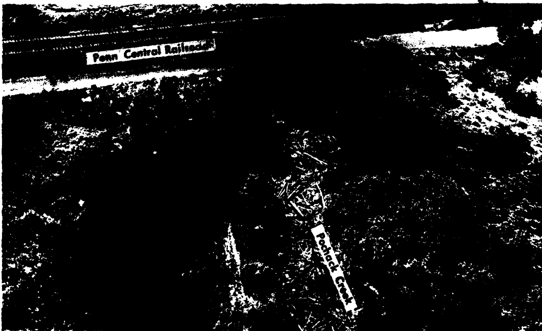
PHOTOGRAPH 9. Channel capacity reduced by debris deposited by tide in Pochack Creek at Penn Central railroad tracks (looking upstream). Condition illustrated is typical of tidal reach of all streams in study area. (August 1968.)
