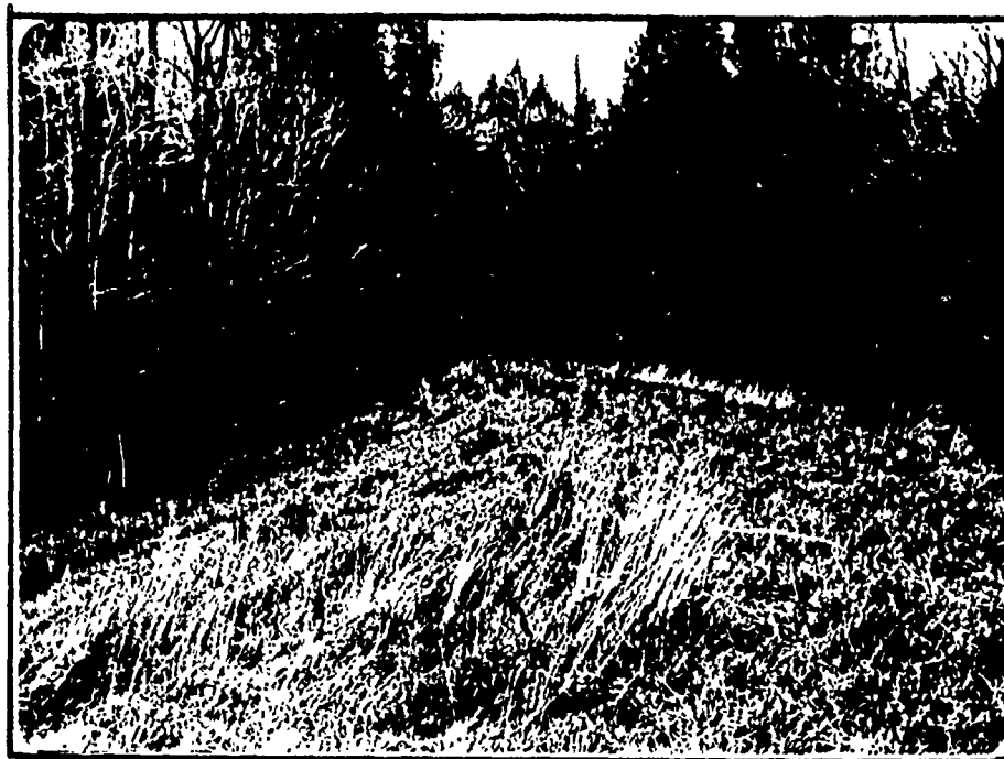
VIEW TO LEFT END OF EMBANKMENT - NO. 2
