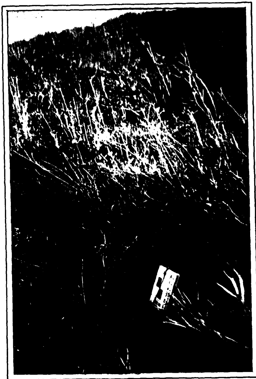
DAMAGE TO SLOPE NEAR WATER LINE, PROBABLY CAUSED BY FOOT TRAFFIC.
