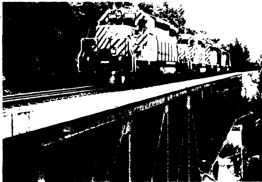
RECORDINGS OF STRAIN WERE TAKEN WHILE BRIDGE WAS LOADED WITH A MOVING FREIGHT TRAIN
