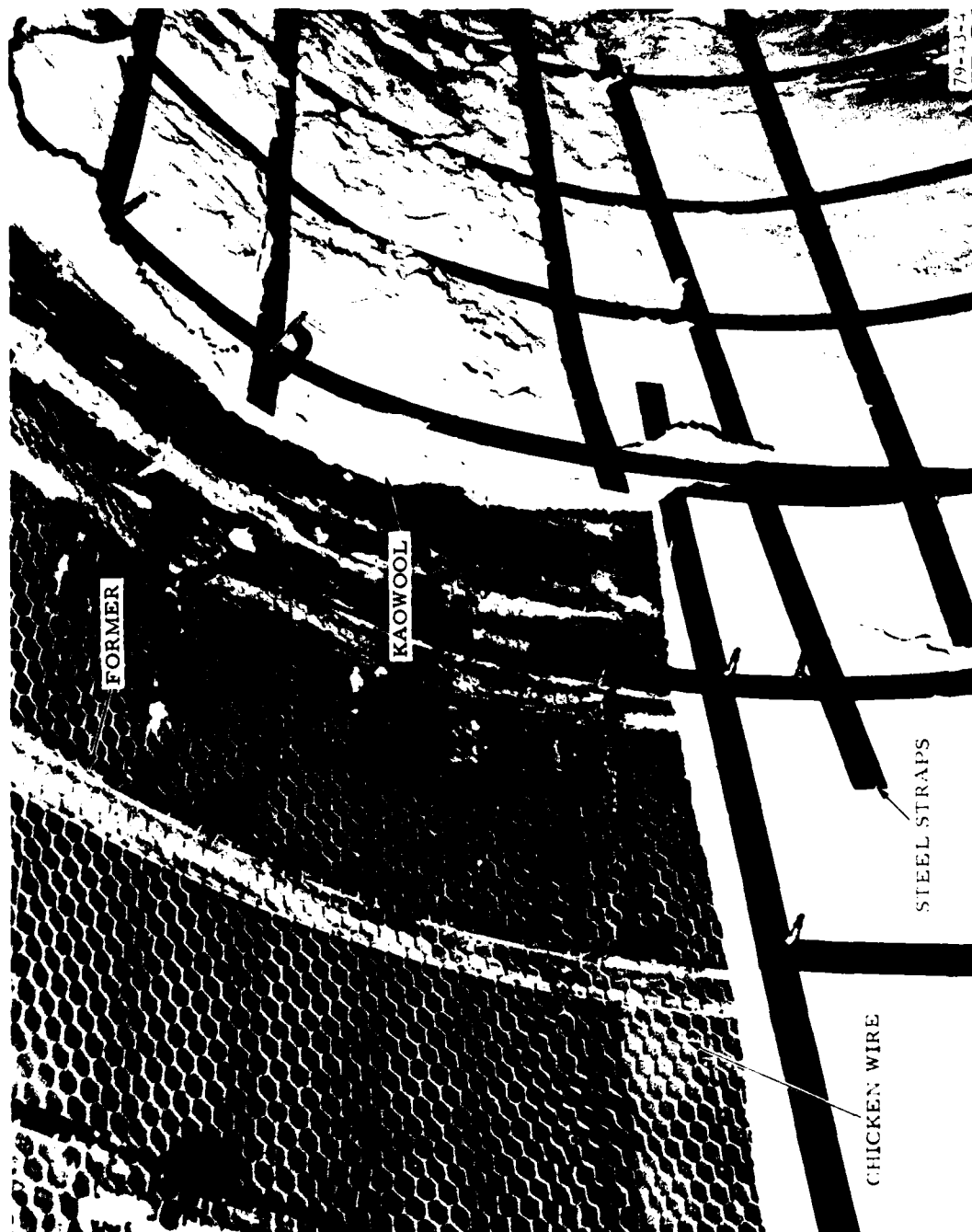
FIGURE 4. CONFIGURATION OF THE FIRE-HARDENED AREA
