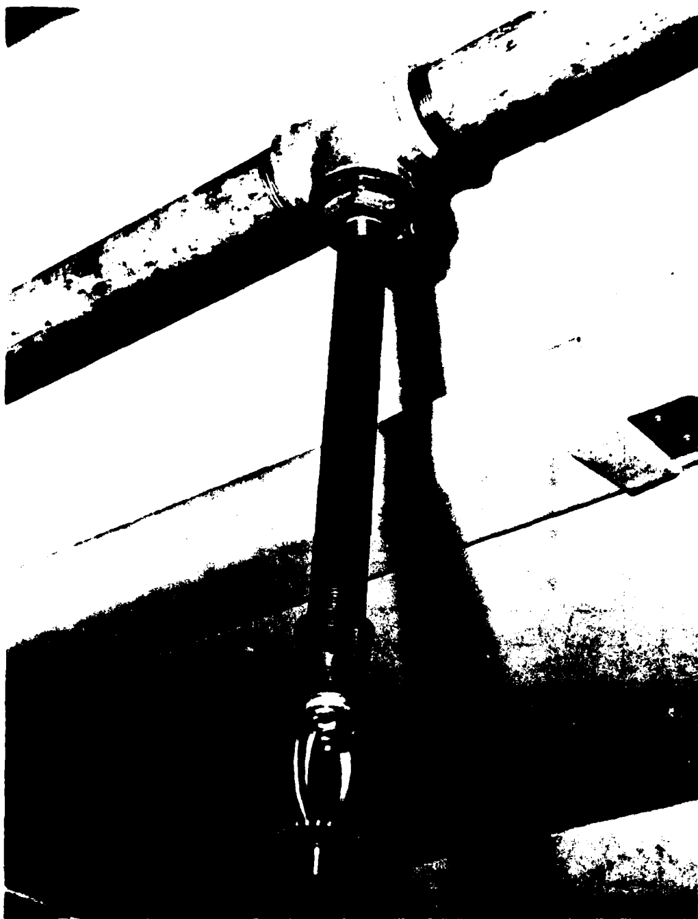
FIGURE 5. FOAM-WATER (AFFF) SPRINKLER HEAD
