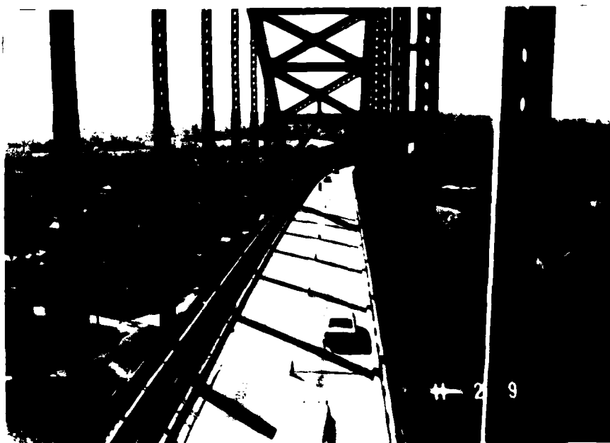
Photograph 2 - Roadway view, looking south through arch span.
