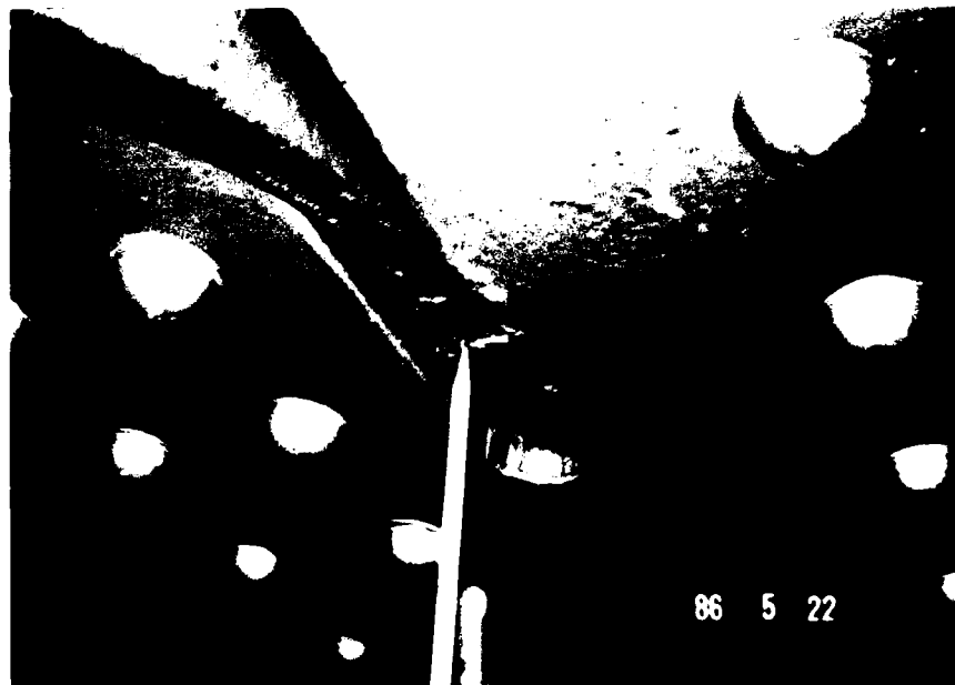
Photograph 17 - Crack in east gusset plate of east truss of tied arch at Panel Point U6.
