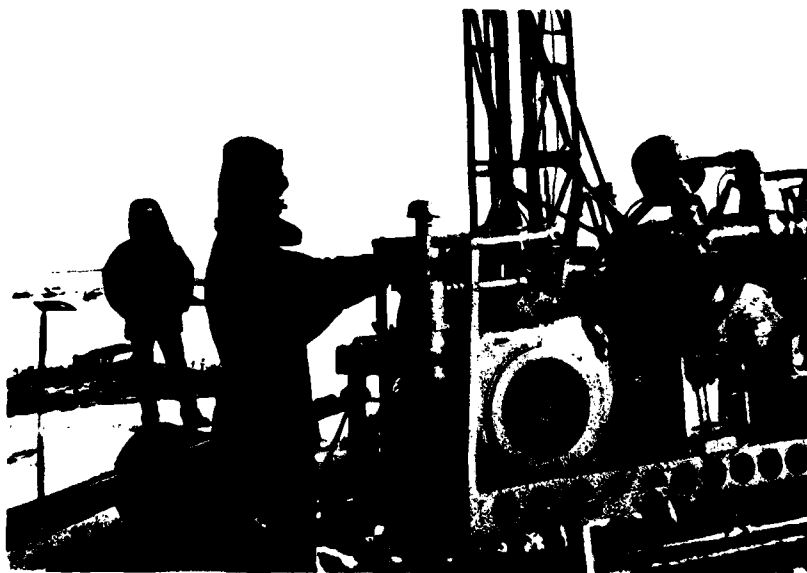
Figure 10. Warming the core barrel on the air compressor manifold.
