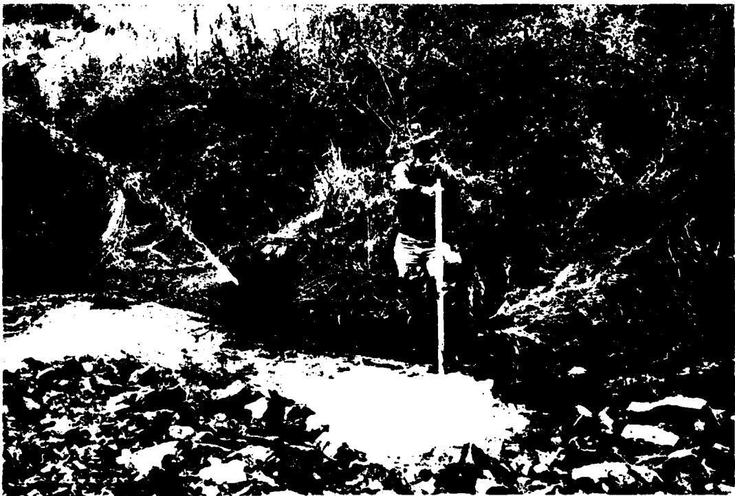
PHOTO 4. Principal Outlet (Marked by Rod) and Emergency Drawdown Outlet
