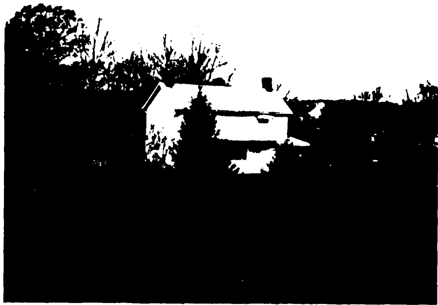
PHOTO 12. INHABITED RESIDENCE DOWNSTREAM OF DAM
