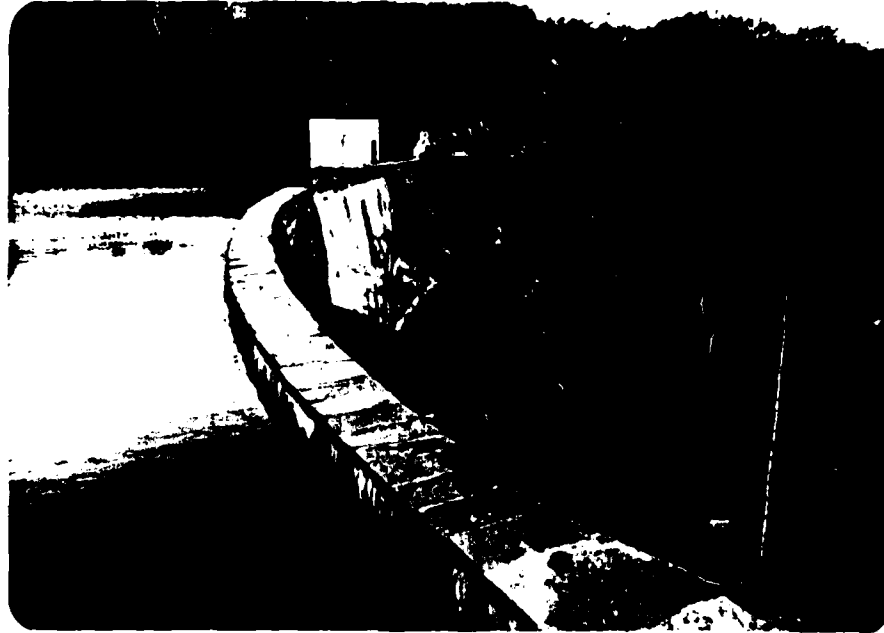
A. View From Right Abutment
