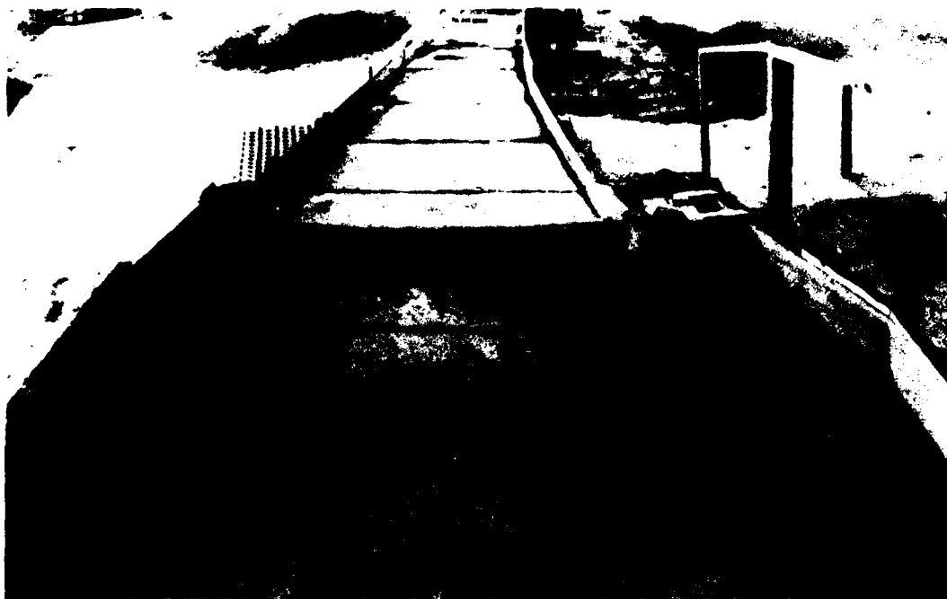
Photo 7. Looking downstream at the type 3 curved wing wall on the right abutment of Westvaco Dam
