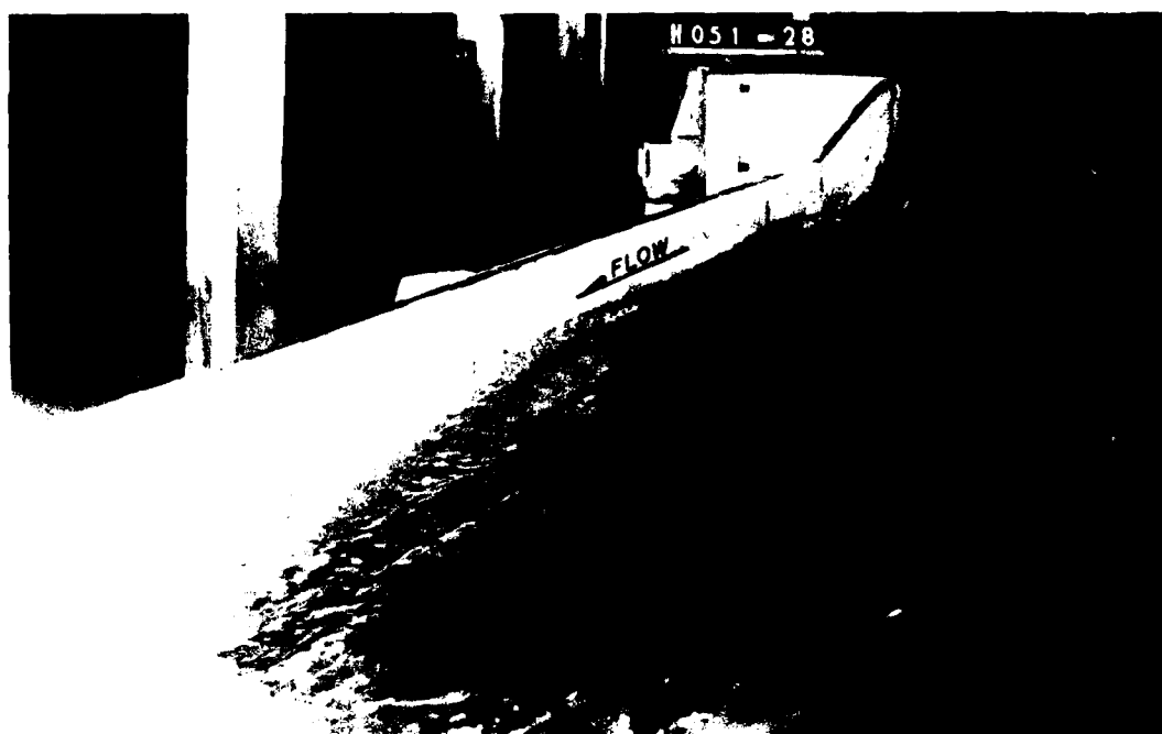
Photo 3. Looking upstream at the right side of Westvaco Dam showing the drawdown in the water surface at the right abutment; discharge 13,400 cfs
