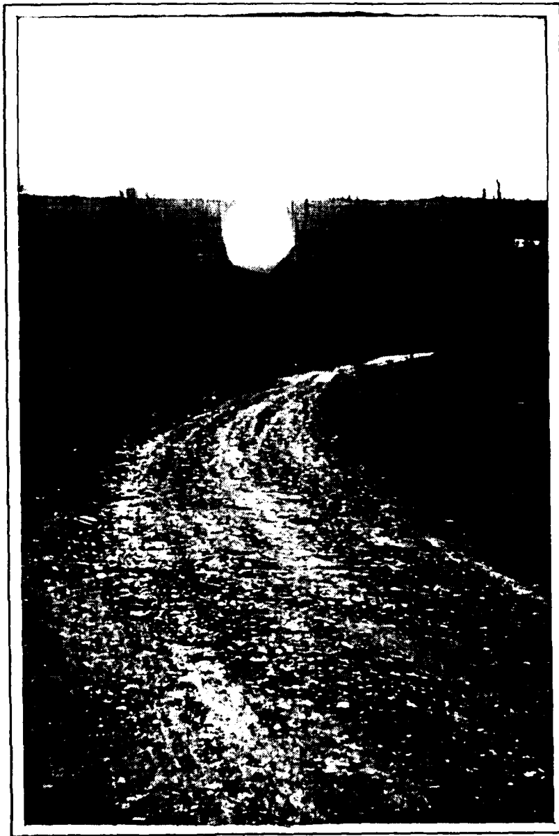
ROADWAY OVER DAM. GRAVEL WAS RECENTLY ADDED TO A LOW SPOT.
