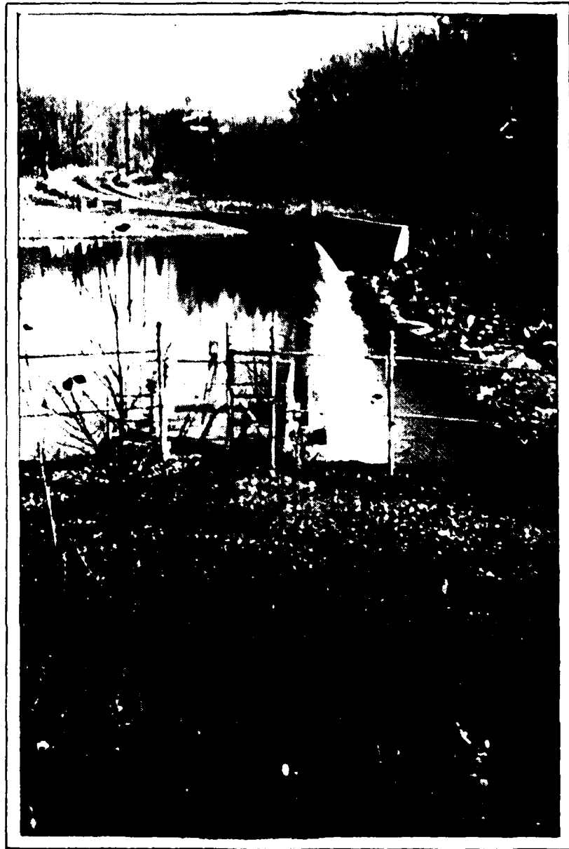
KNIGHTS LAKE DAM, 600 FEET BELOW DEEP CREEK DAM.
