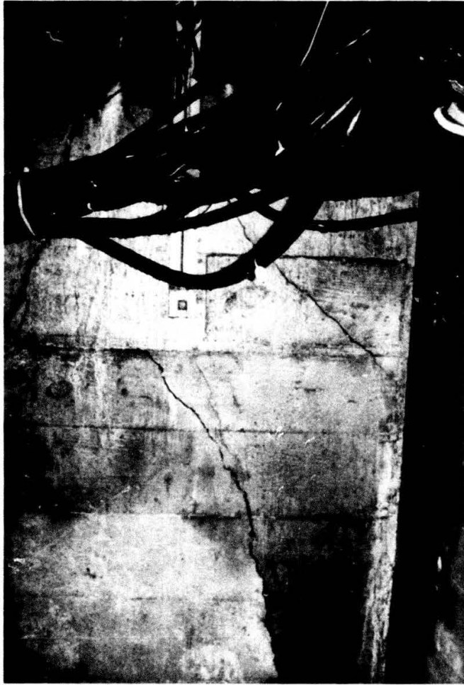
Figure A3. Upstream face at lockside turn of river wall, cable gallery, monolith 11
