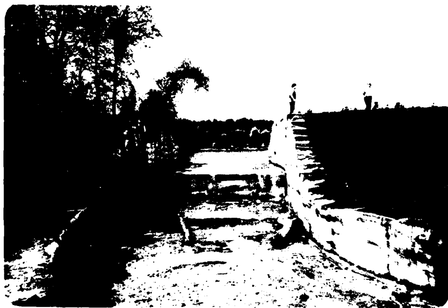
Auxiliary spillway crest - looking upstream
