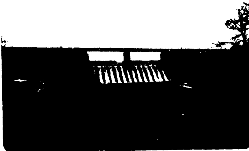
OVERFLOW SPILLWAY AND ABUTMENTS
