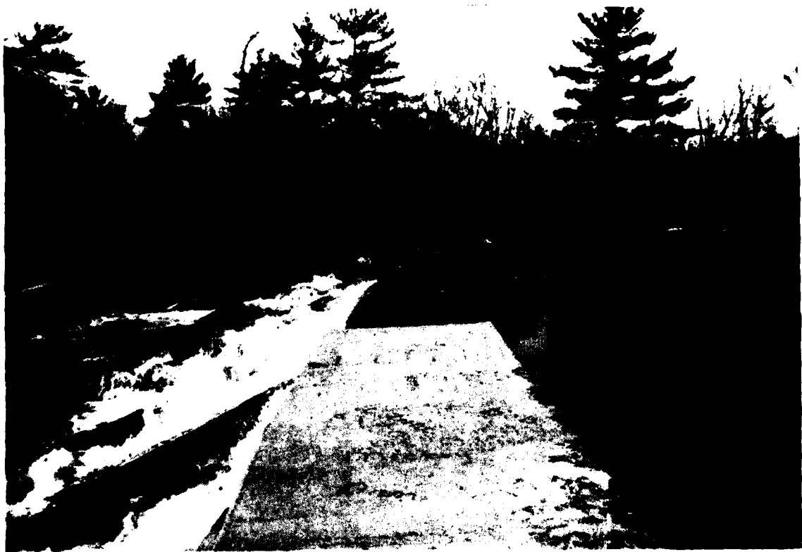
Overview of dam spillway looking north. Spillway caps bedrock providing reservoir area above rapids.
