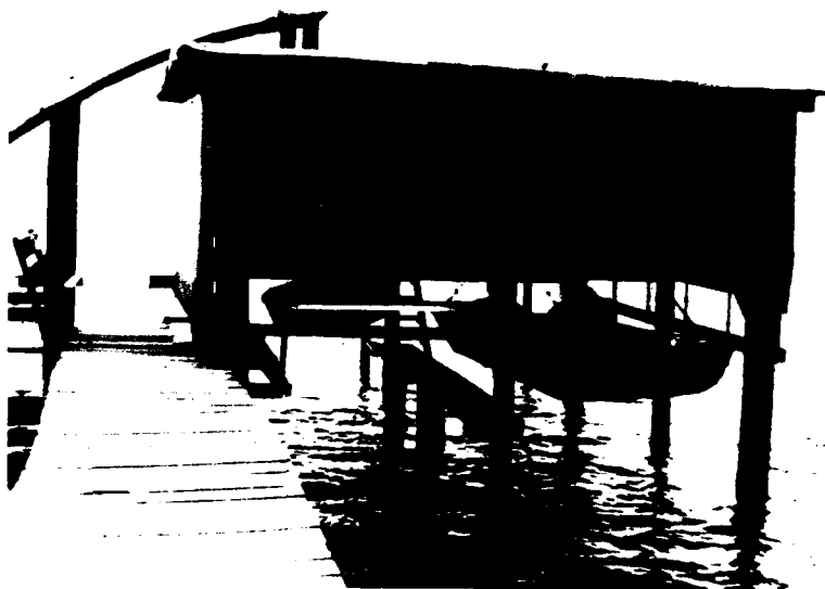
Boathouse with Boats Suspended in Hoist
