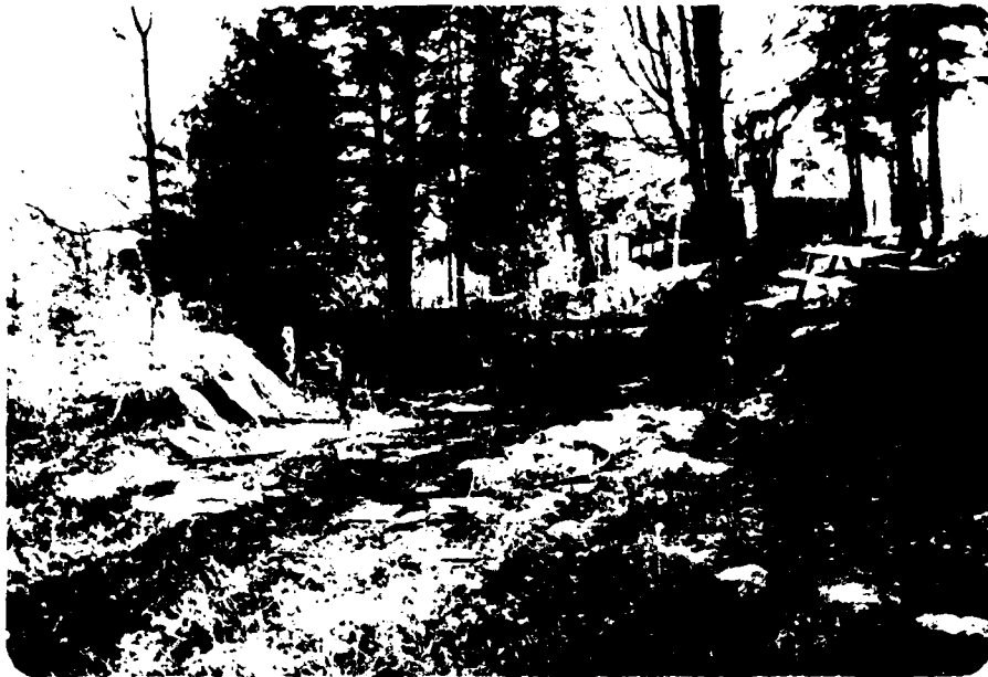
Crest of Auxiliary Spillway - Note Wood Framework Across Inlet
