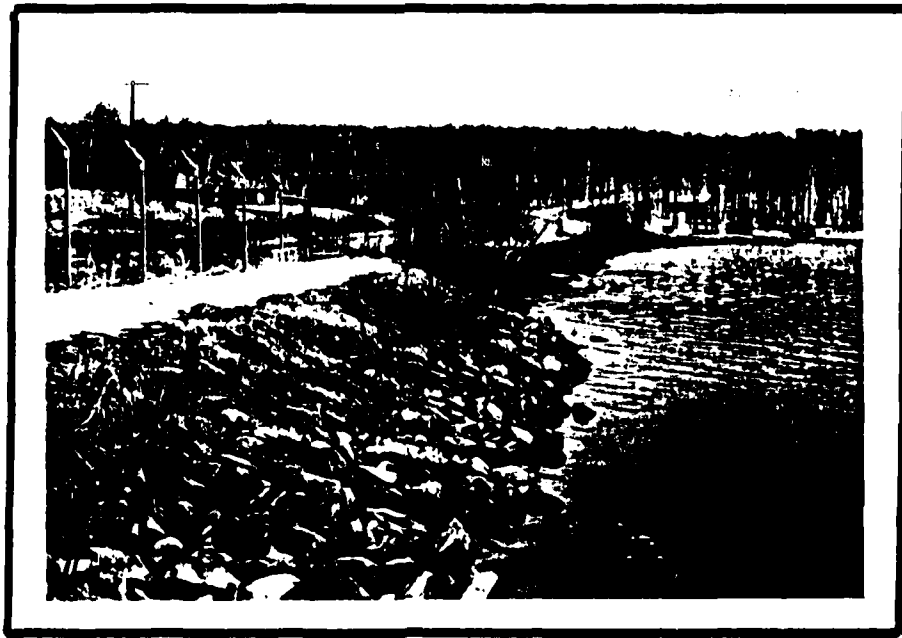
UPSTREAM SLOPE - NO. 3
