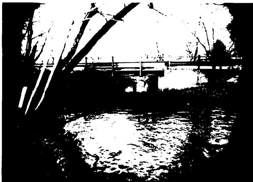
Photo 9 - View of roadway bridge (Upper Greenwood Road) crossing over channel approximately 200 feet downstream from the spillway.
