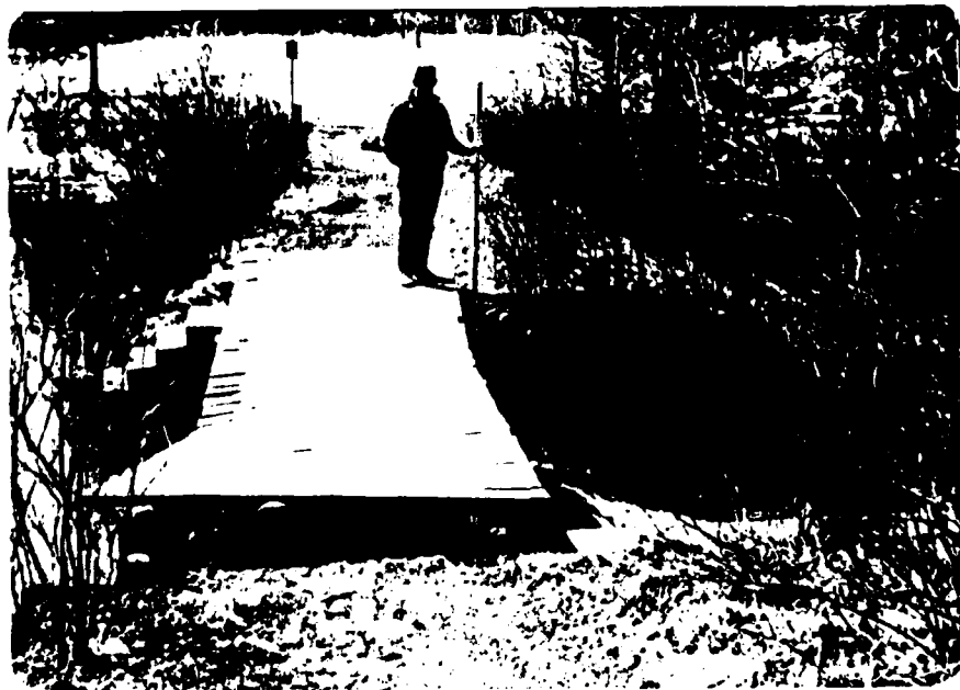
F. Spillway Bridge
