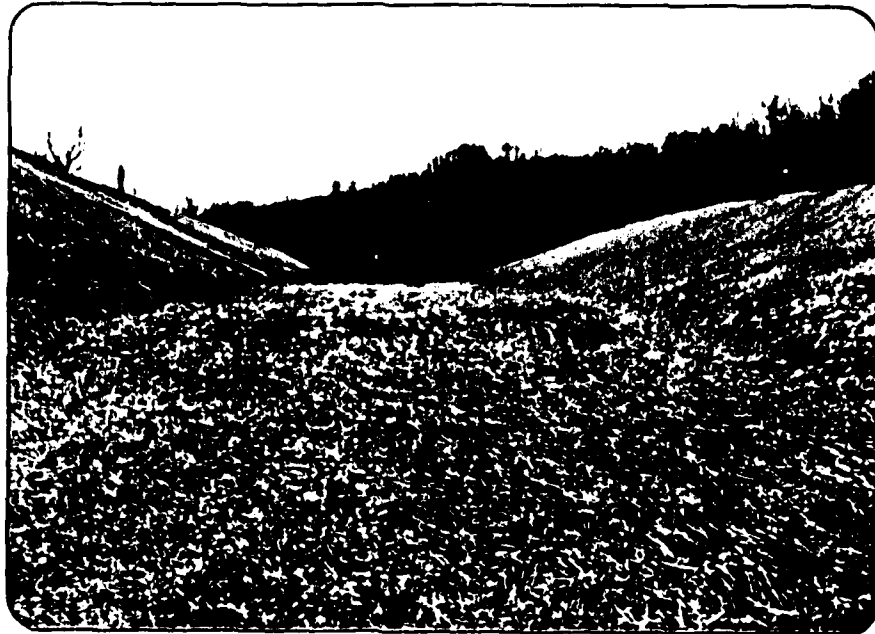
PHOTO 5. View of the Emergency Spillway Looking Upstream
