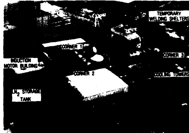
Fig. 21 Aerial view of NTF construction site (2/4/80).
