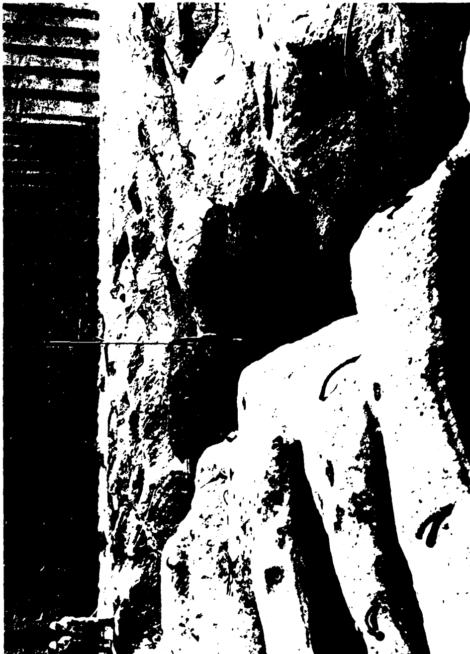
Figure 1. Erosion of stilling basin floor slab, Dworshak Dam
