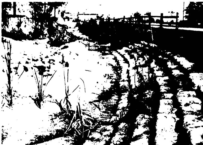
Figure 11. In-place sack revetment. The sacks were fabricated from filter fabric material
