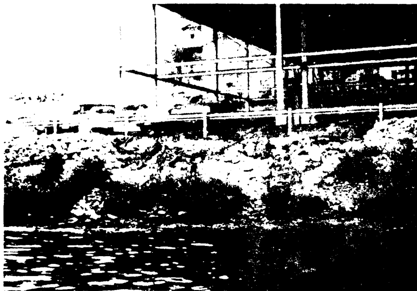
Figure 30. Damage to bank protection at Wheeling Wharf Parking Garage after the 1972 failure. Riprap has slid down the slope into the river and the filter fabric has ripped.
