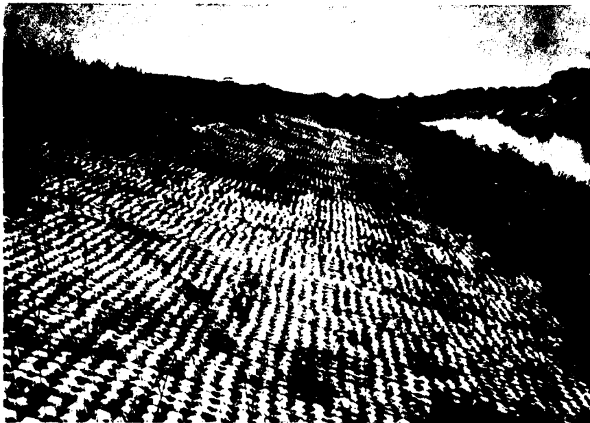
Figure 58. General downstream view of cellular block section of Morameal Revetment, La. (9 May 1978)
