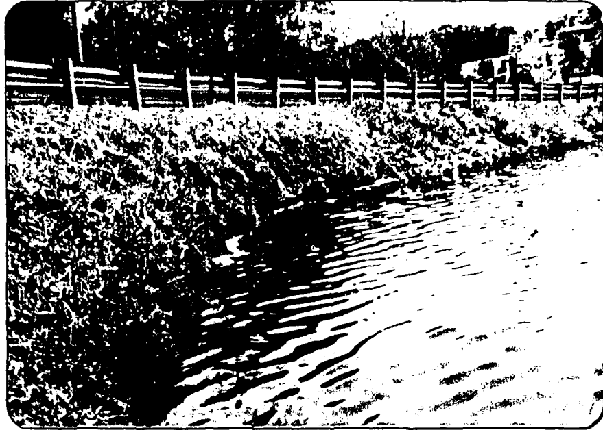
PHOTO 7. View of Erosion along Upstream Face of Embankment
