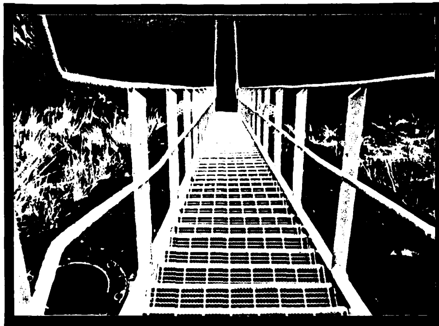
Photo 9 Principal Spillway Intake Ports and access stairway.
