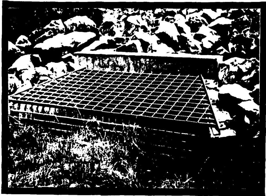
Photo 7 Underflow Pipes Inlet at downstream (up-valley) toe of Embankment B.
