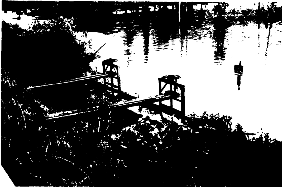
PHOTO 1. Spillway Weir and Controls for Emergency Gates
