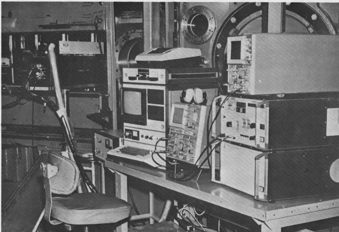
Figure 21. Installation of System in Tunnel A (Mach 4.5).
