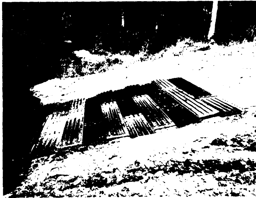
d. Mat sections on slope and in lake prior to anchoring
