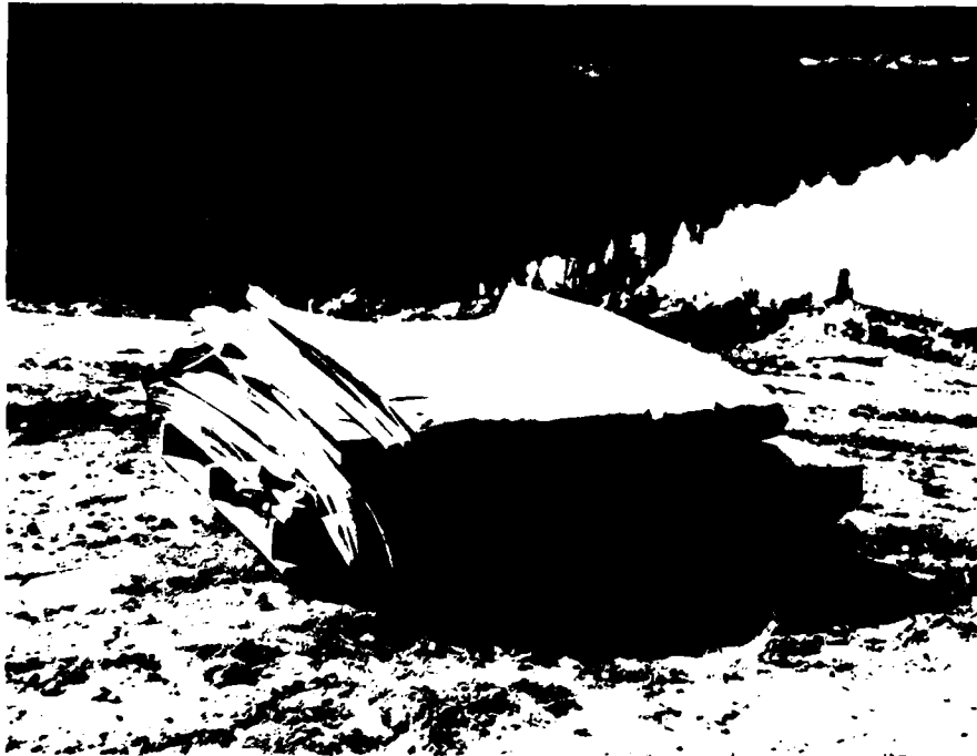
a. Folded 36- by 100-ft T17 membrane as delivered to top of slope
