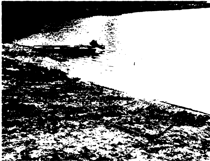
e. Reanchored mat after realignment and reanchoring
