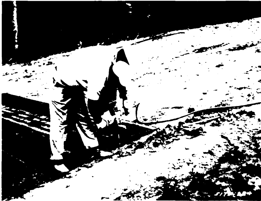
e. Anchor placement to prevent downward sliding into lake
