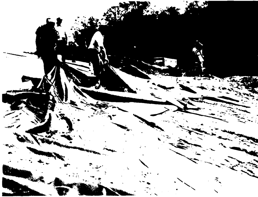
k. Damaged membrane shredded at water's edge by spinning tracks of vehicle
