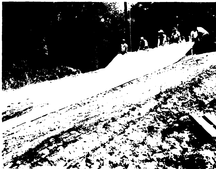
d. Stretching of membrane upslope prior to anchoring
