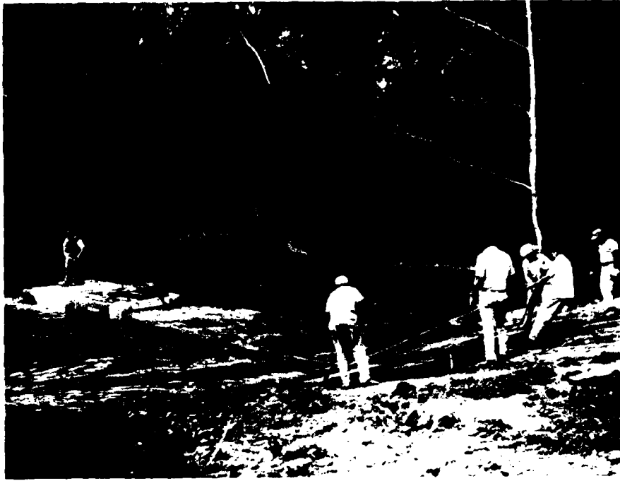
c. Mat sections being dragged by cable into lake
