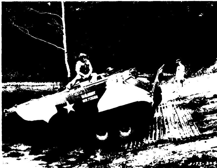
f. M113 APC almost successfully exiting lake (note mat was pulled downslope until "go" condition encountered with mat located as shown in Photo 5g)
