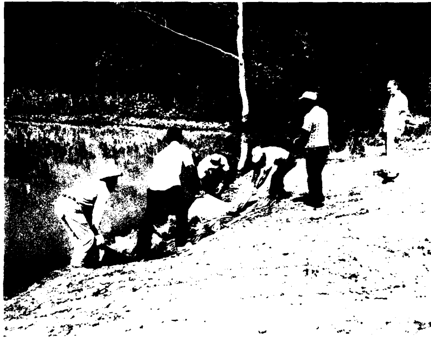
c. Lateral unfolding procedure to place membrane across slope
