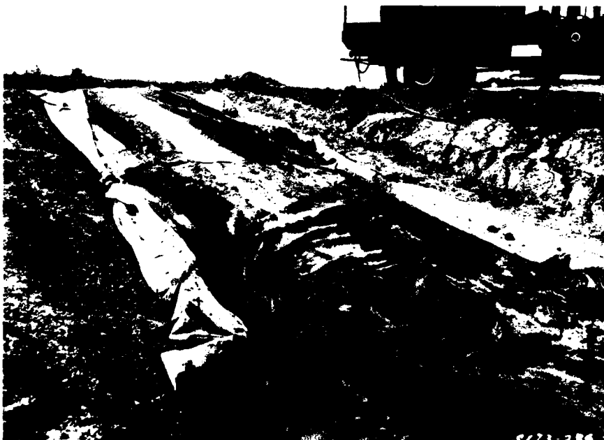
b. View of membrane and dry slope after vehicle traffic
