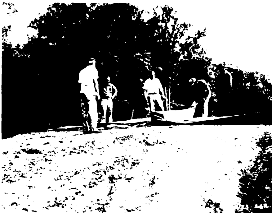
b. Lateral unfolding of membrane across width of slope
