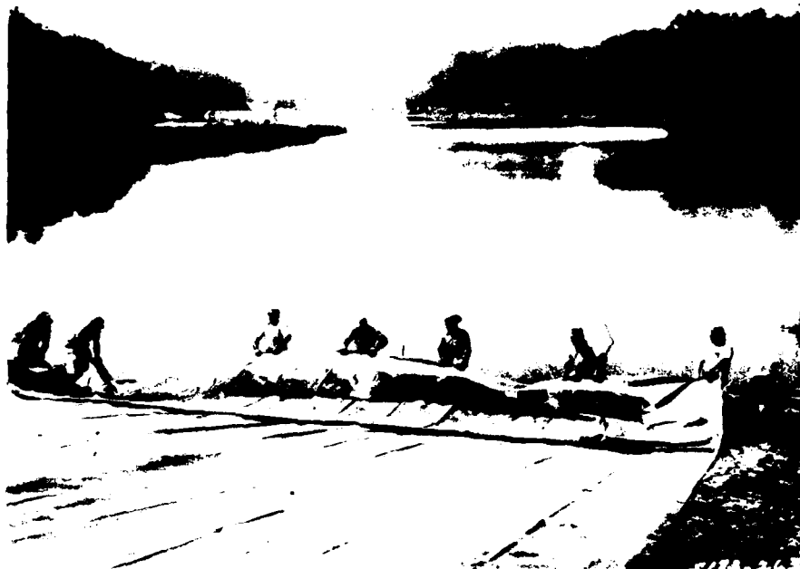
c. Pulling of membrane downslope prior to anchoring
