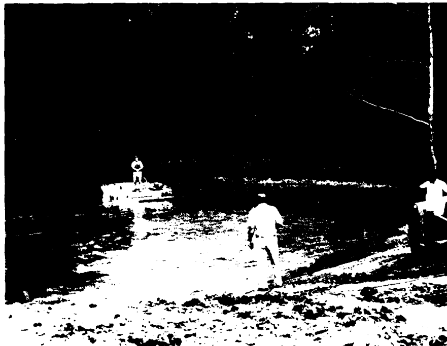
d. Sandbag anchors being placed in lake (note one entangled line being freed by WES personnel)
