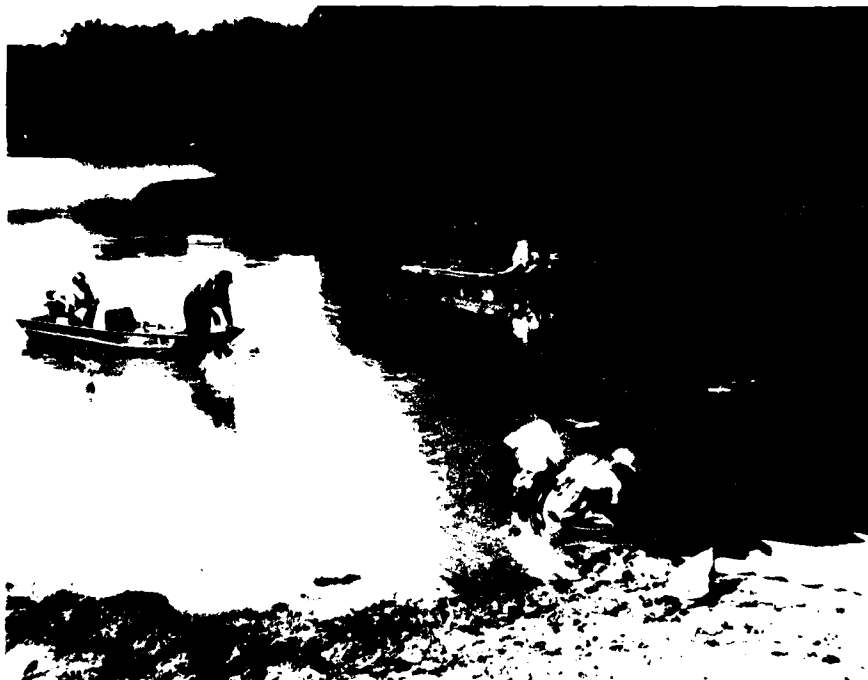
f. Cable and sandbag anchoring of membrane in lake
