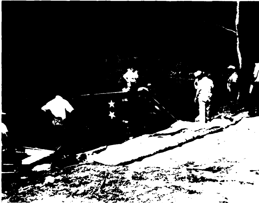
e. Membrane placement into lake underwater
