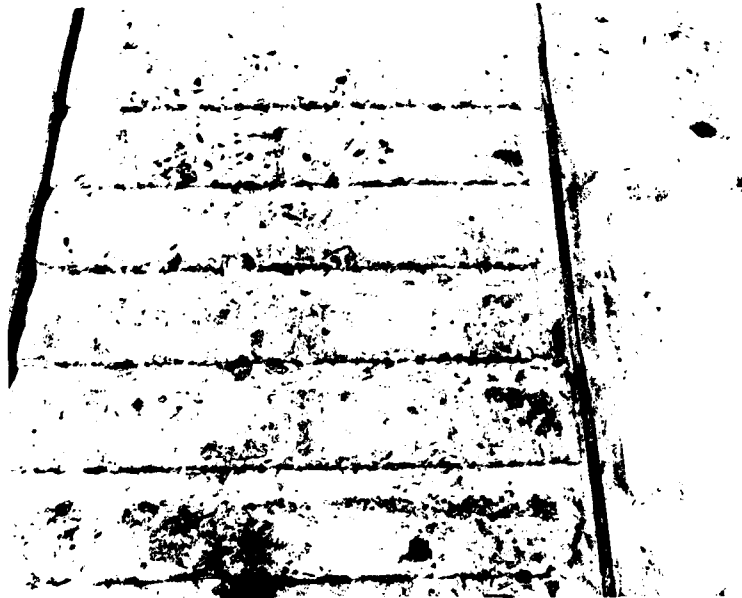
3 GROOVES PRODUCED BY REFLEX-PERCUSSIVE PROCESS
